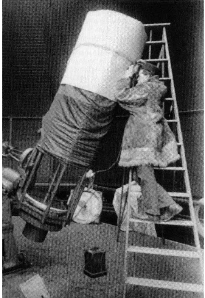
Anyone with a large Dobsonian can immediately identify with this photo. A 24 inch f 4-ish truss tube telescope with a cloth shroud (note the front end extension, which I imagine is black on the inside) and with the Newtonian focus accessible with a ladder is not unusual today. A scope this size is probably mounted as a Dobsonian today, but then it's also more likely to have a goto drive too.
